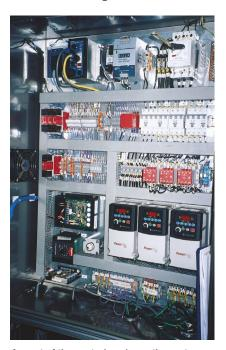
As part of the control package, the system integrator wrote the control logic for the entire system utilizing DeviceNet communication protocol, which, in this case, allows communication with 200 I/O points.
